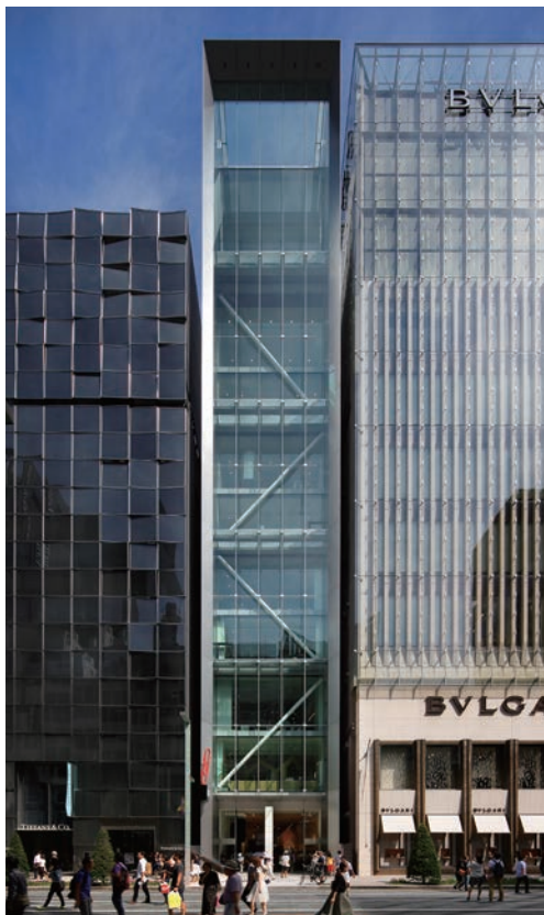
店舗外観 / Exterior View of the store
